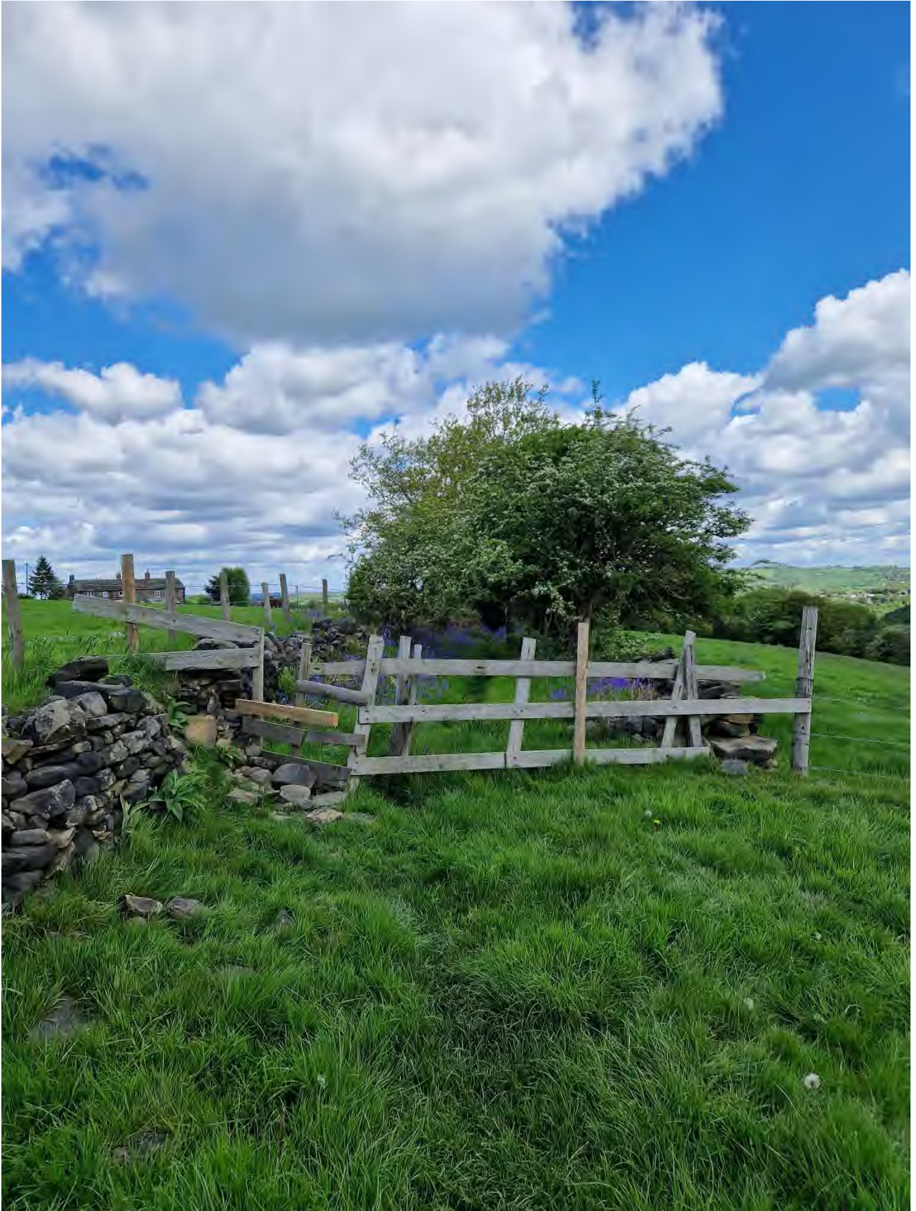
Photo 17: Close-up of third wooden stile structure.
